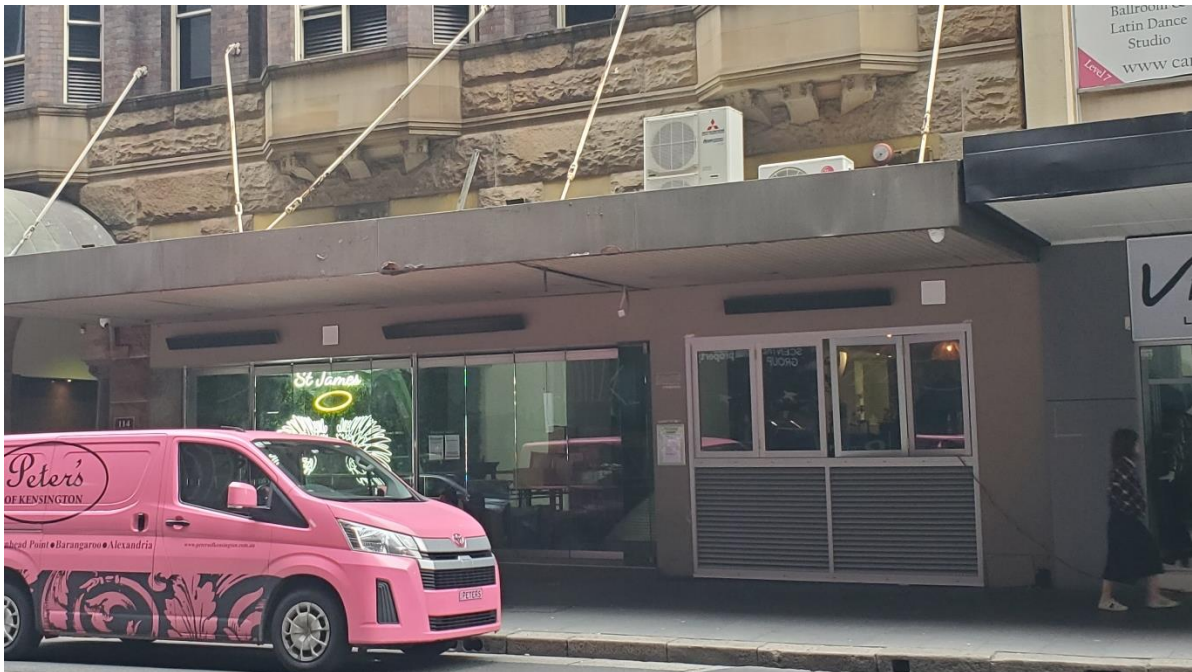
Figure 4: Ground floor view of subject site from Castlereagh Street
