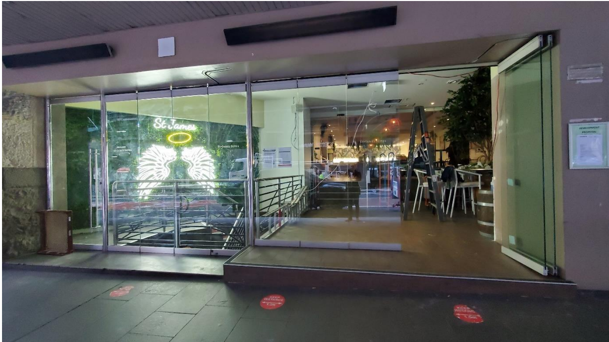
Figure 7: External view of site entrance fronting Castlereagh Street
