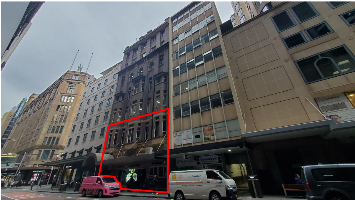
Figure 2: Subject site context from Castlereagh Street- subject site in red with 122 Castlereagh Street directly to the right and 83-87 Market Street directly to the left
